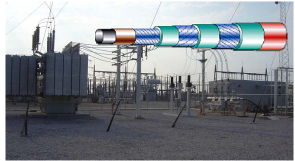
AEP Columbus superconducting cable. Inset is a schematic of the innovative triaxial cable design with concentric superconducting layers
