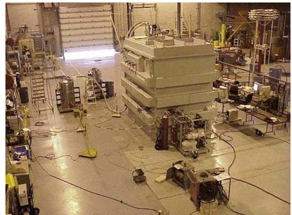
Demonstration superconducting transformer
